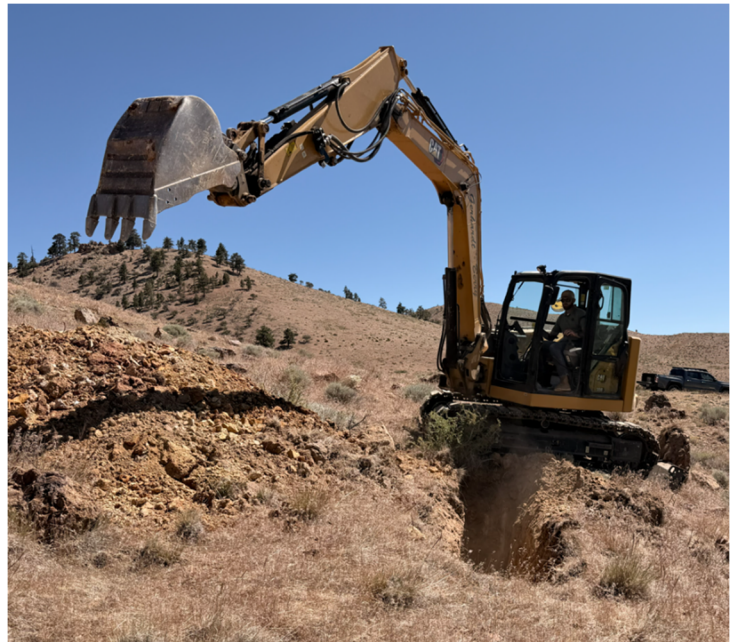
Test Pit Exploration
